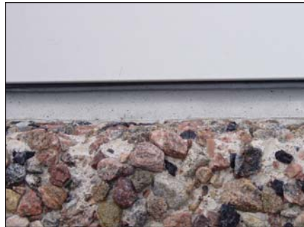
Do not carry exposed aggregate finish beyond window interface.
