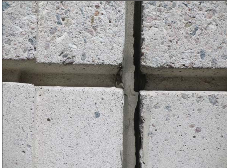
Precast remained clean, sealant has retained atmospheric dirt.
