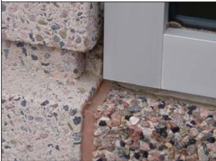
Do not carry exposed aggregate finish beyond window interface.
